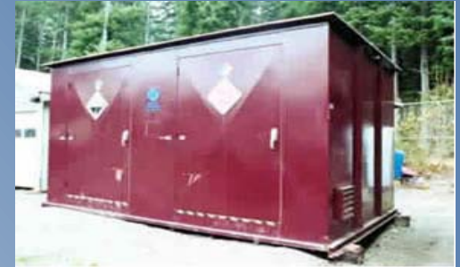
Waste Storage Unit
